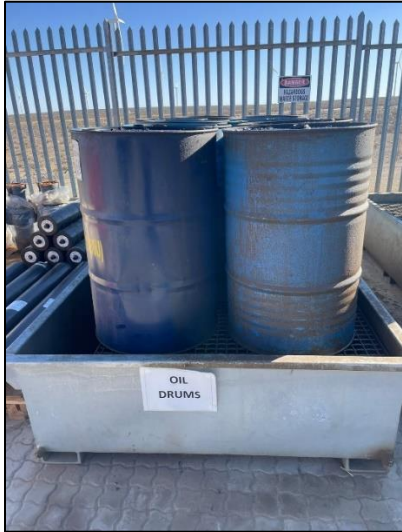
13. Used oil in secondary containment to contain leaks
