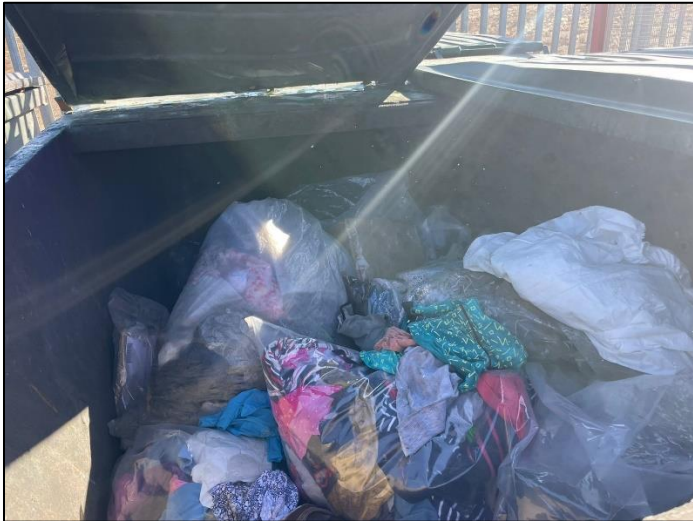
11. Oily rags and hazardous waste stored in skips with lids until removal from site
