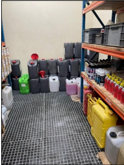
5. Built-in bund within the chemical store
